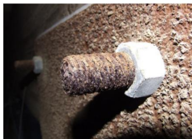
Fig. 1. Corrosion of metal structures
